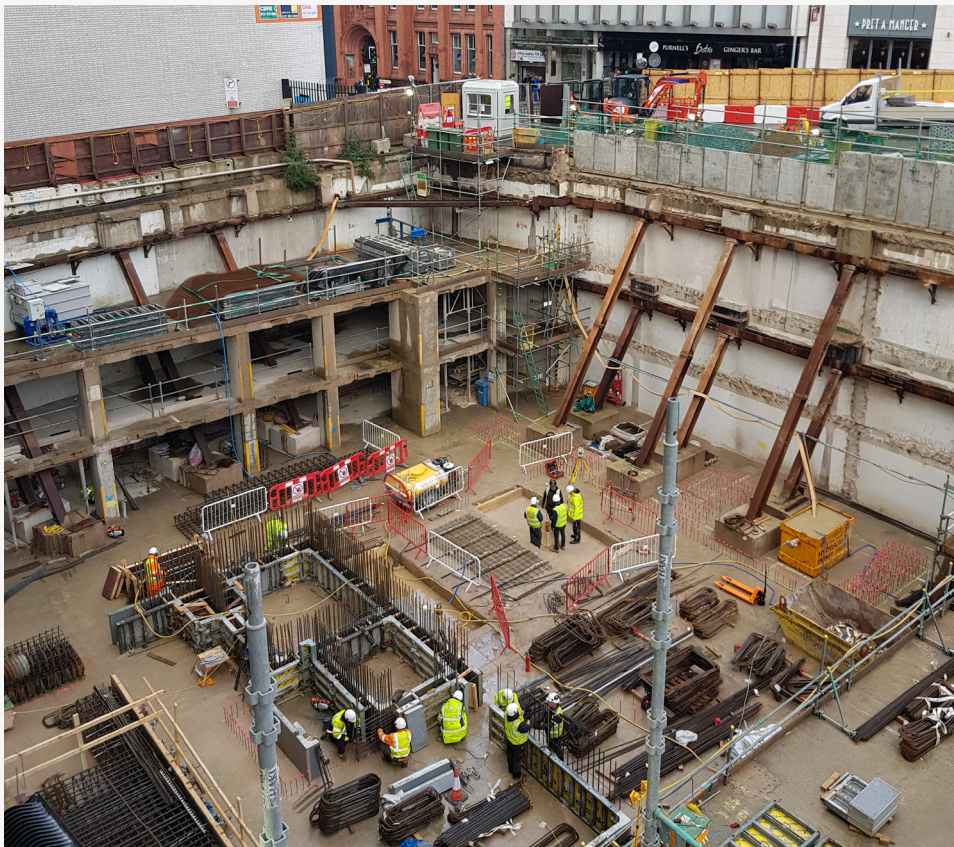
Structural Engineer: Davies Maguire
